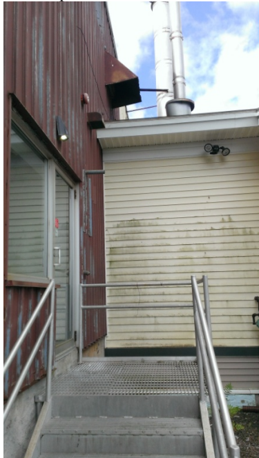
LED replacement fixtures
