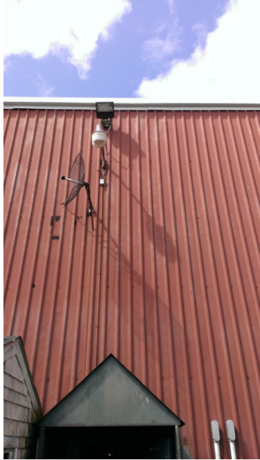
Varying fixtures on east wall
