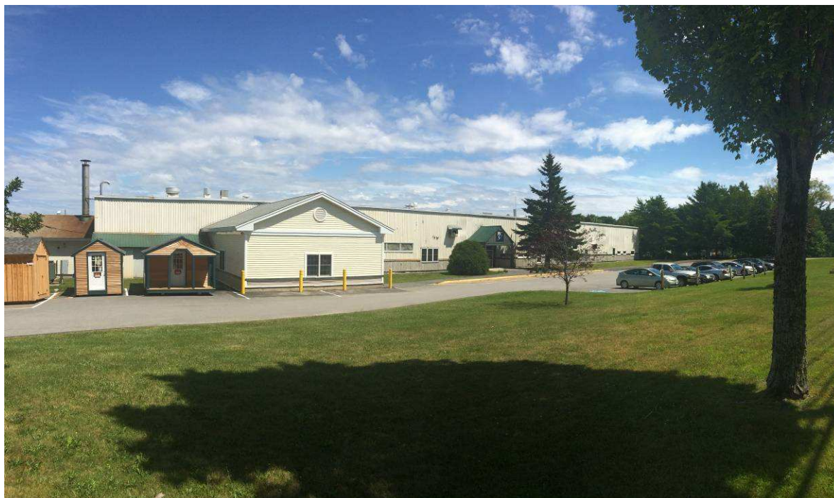
Photo 1: General view of Midcoast School of Technology from Route 73.
